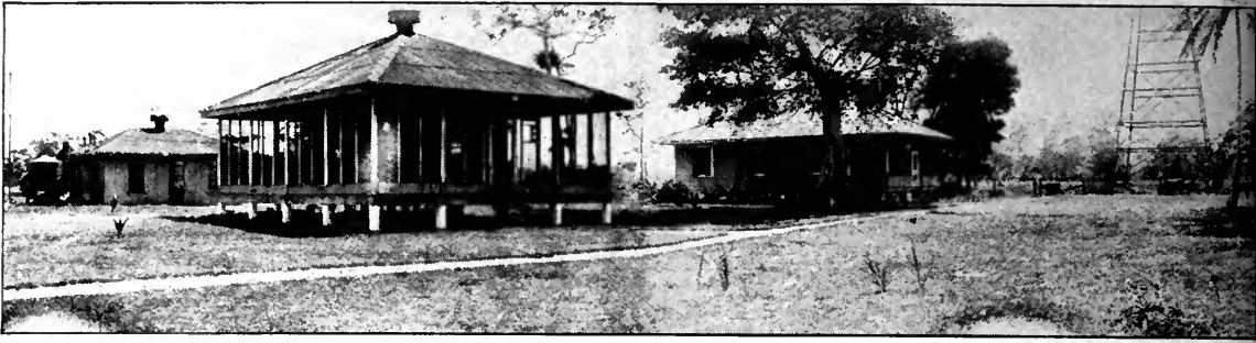
THE RADIO STATION AT TELA, HONDURAS
